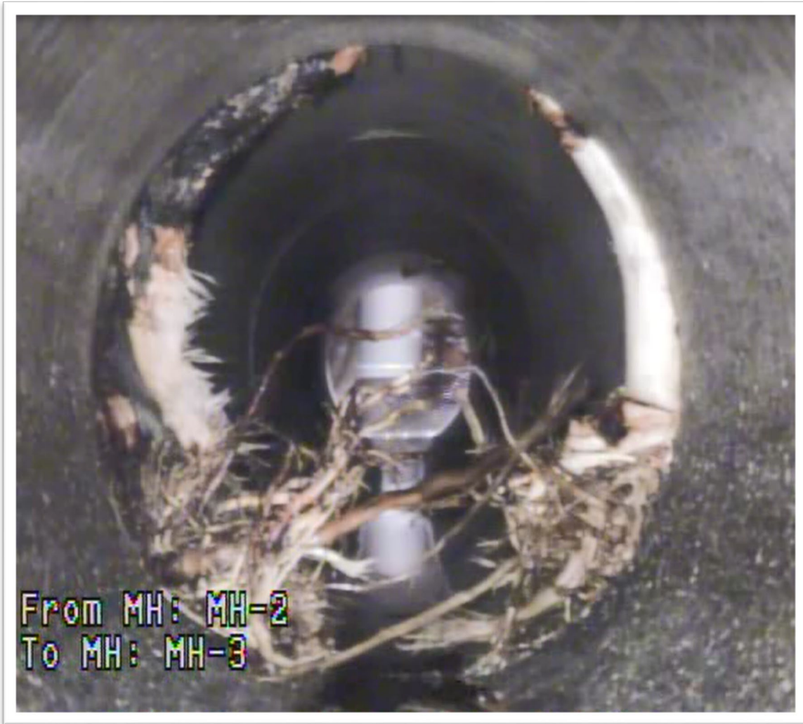
Storm Drain Root Intrusion
